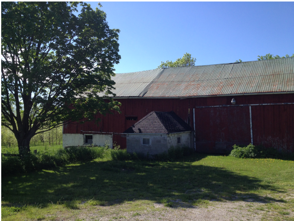
Photo No. 4: Agricultural barn on-site, June 2021
