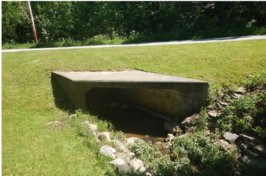
Figures 17 & 18: Culvert with BCI rating of 75
