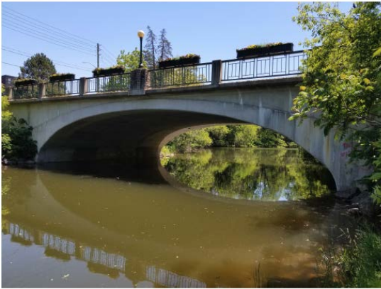
Figures 15 & 16: Vehicular Bridge with BCI rating of 82
