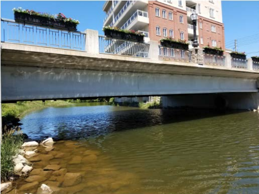
Figures 13 & 14: Vehicular Bridge with BCI rating of 100
