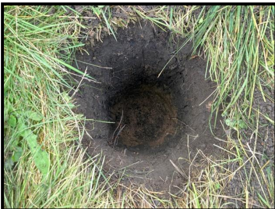
Image 9: Test Pit Survey (August 5, 2021; Facing North)
