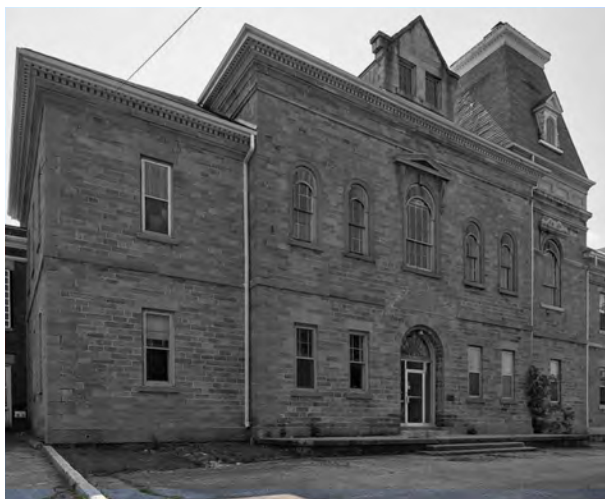
Figure 9: Courthouse, Existing Front Facade
