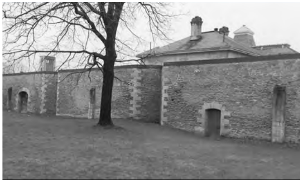
Figure 39: Rear Yard, Jail Yard Walls West Facade
