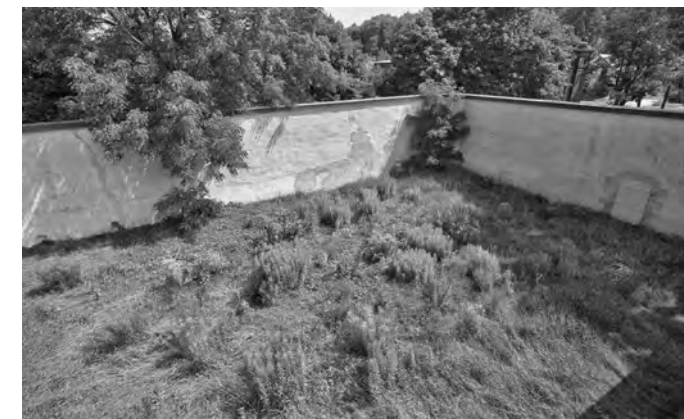
Figure 25: North Jail Yard - Existing
