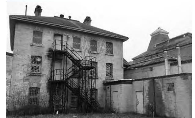
Figure 31: Jail (1869-1877), Existing North Facade
