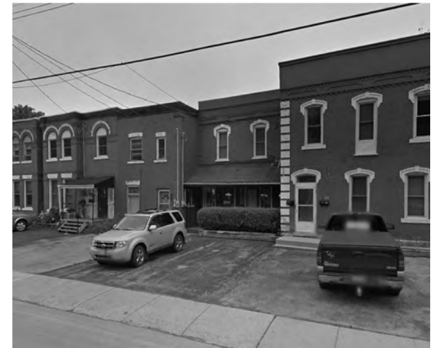
Figure 5: Historic rowhouses along 4th Ave E
