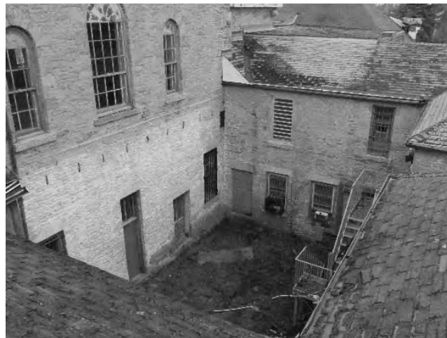
Figure 17: Jail (1854), Existing interior Courtyard
