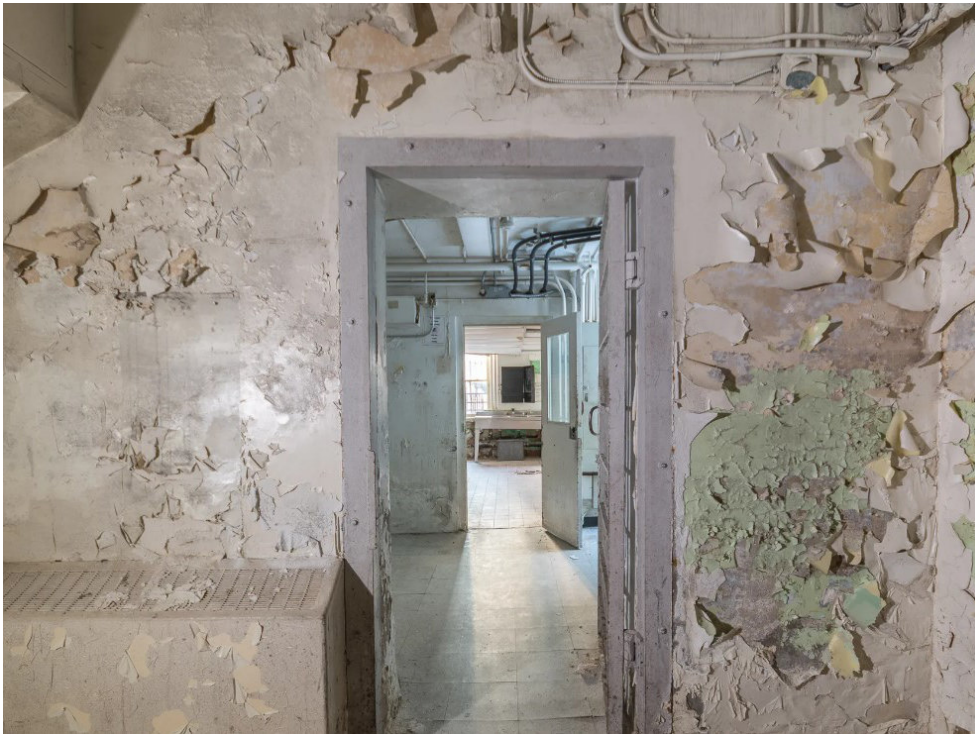
Figure 6.39 Interior view of the Jail Building View of the kitchen entrance.
