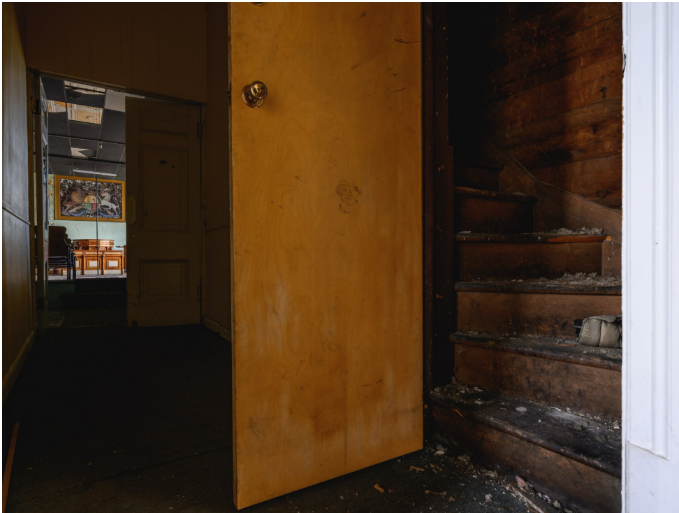
Figure 6.21 Historical Courthouse Staircase to the tower.
