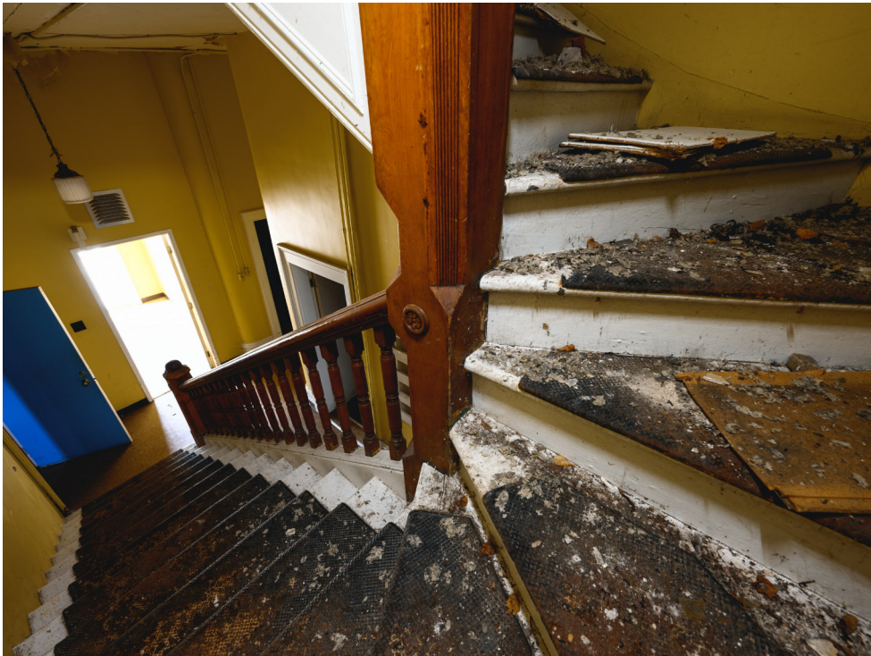
Figure 6.19 Historical Courthouse Detail of the main staircase.
