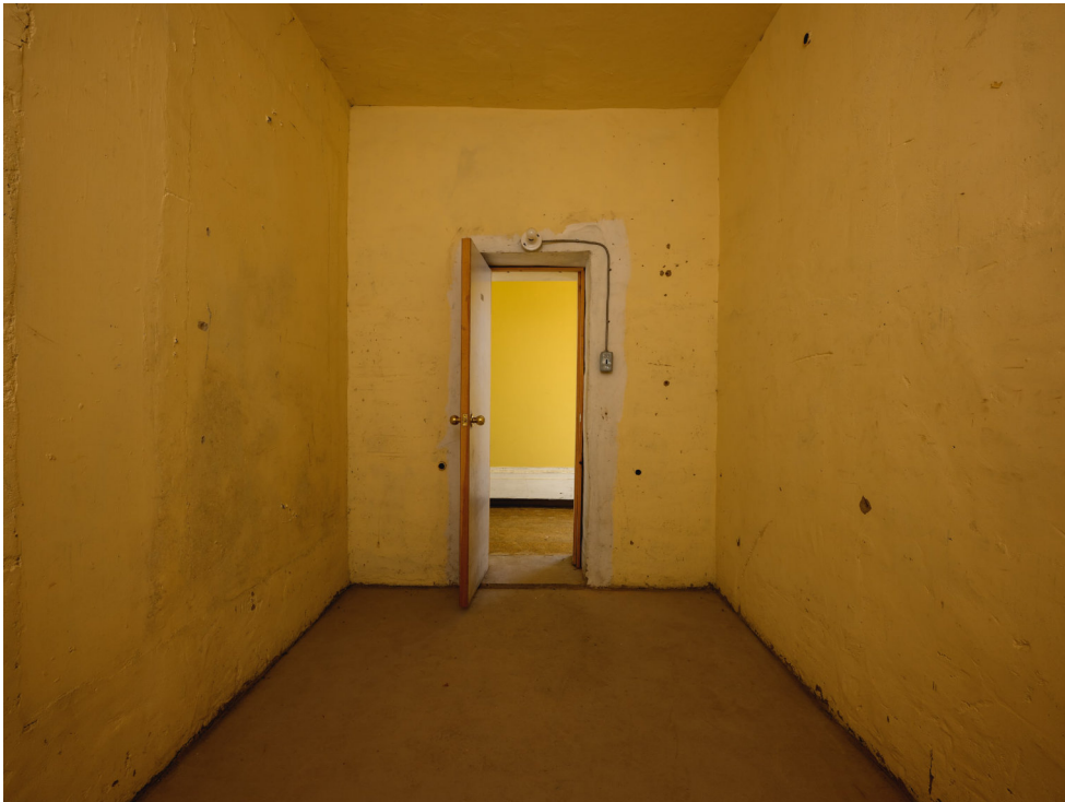
Figure 6.11 Historical Courthouse Ground Floor - Existing Conditions.
