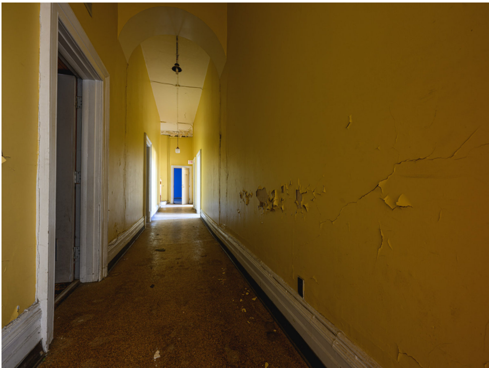
Figure 6.12 Historical Courthouse Ground Floor - Existing Conditions.
