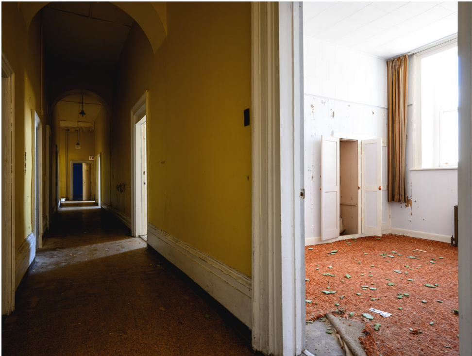
Figure 6.5 Historical Courthouse Ground Floor - Existing Conditions.
