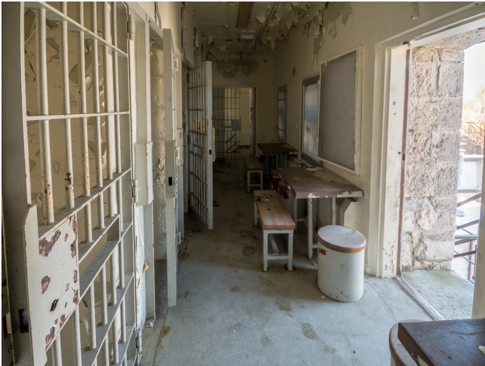
Figure 6.43 Interior view of the Jail Building Access to exterior fire stairs.
