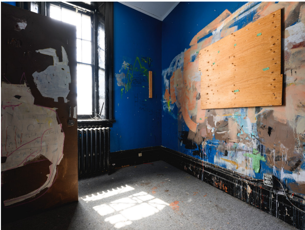
Figure 6.14 Historical Courthouse Ground Floor - Existing Conditions.
