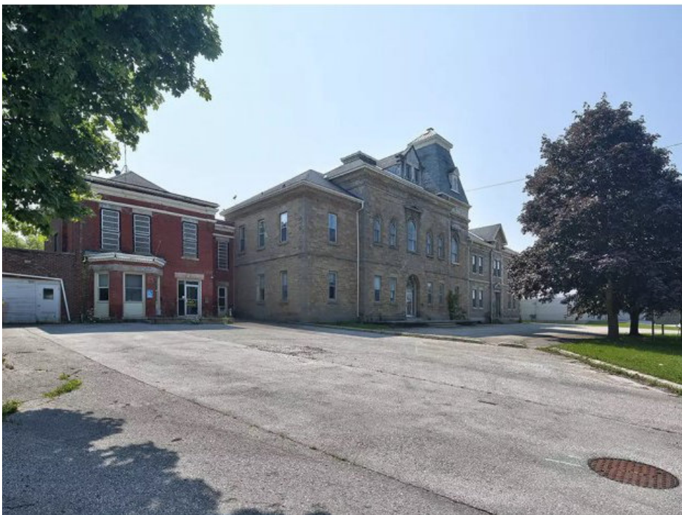
Figure 6.2 Approach to the property from 3rd Avenue.
