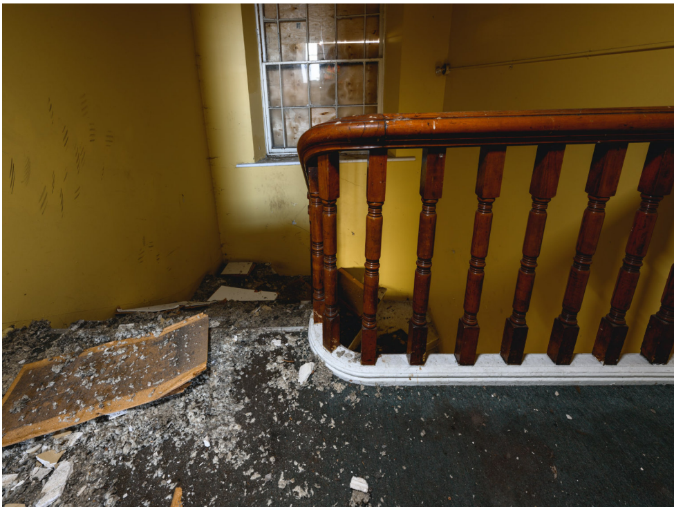
Figure 6.20 Historical Courthouse Detail of the main staircase.
