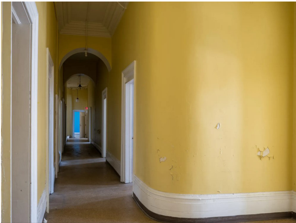
Figure 6.8 Historical Courthouse Ground Floor - Existing Conditions.
