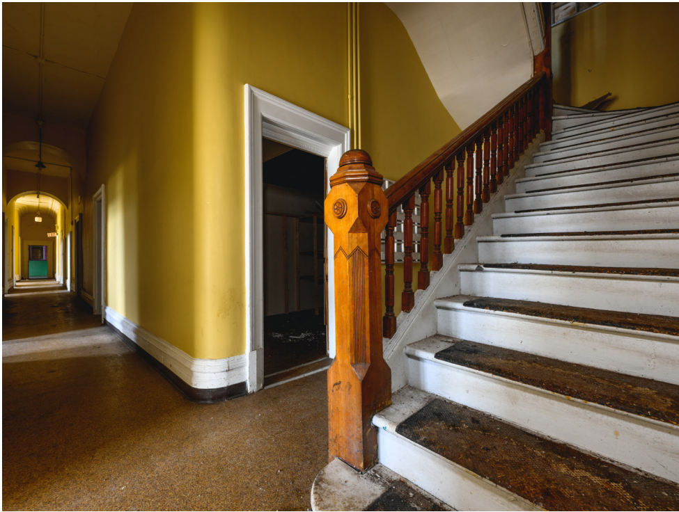
Figure 6.17 Historical Courthouse Ground Floor - Existing Conditions.
