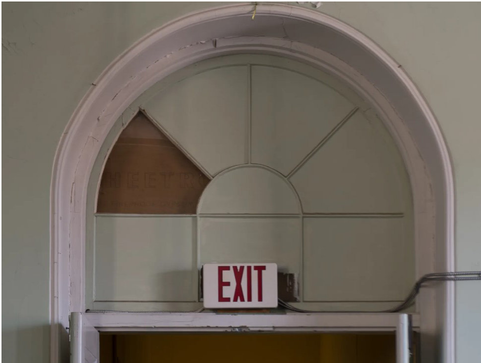
Figure 6.31 Historical Courthouse Detail of interior door opening.
