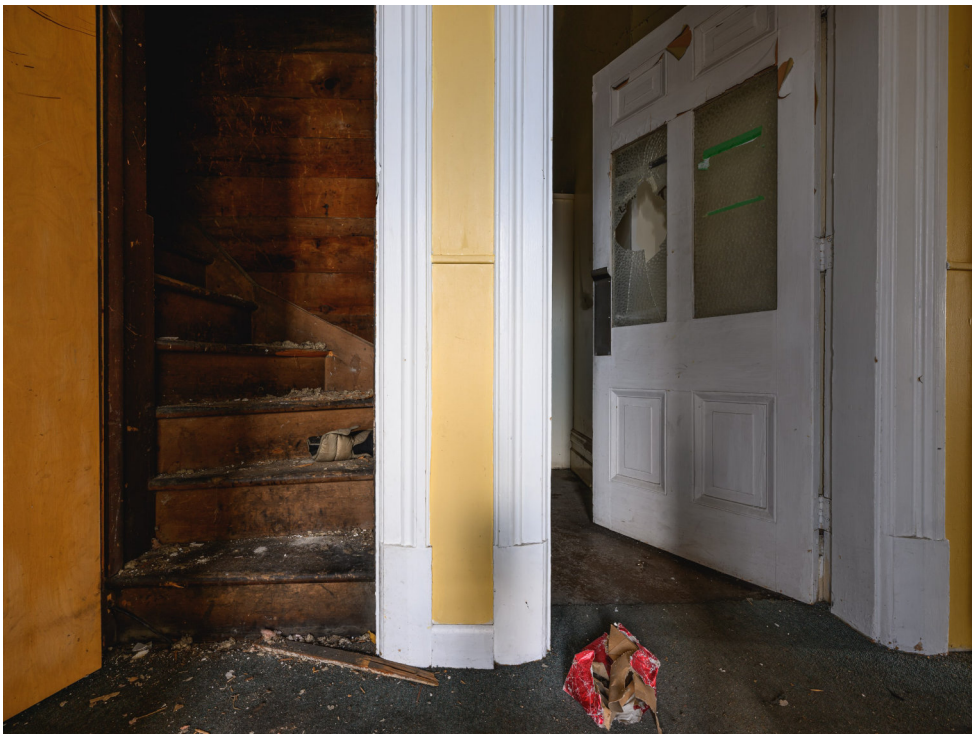
Figure 6.16 Historical Courthouse Ground Floor - Existing Conditions.
