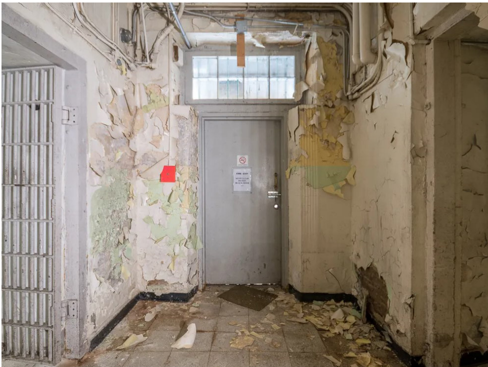
Figure 6.38 Interior view of the Jail Building Ground floor entrance.
