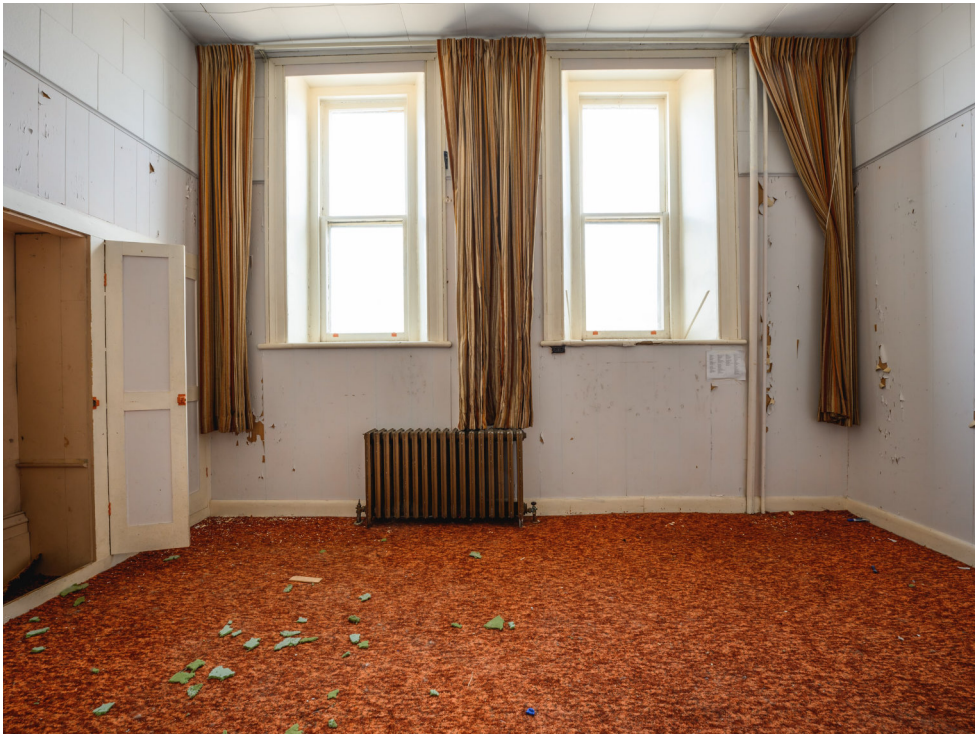
Figure 6.9 Historical Courthouse Ground Floor - Existing Conditions.
