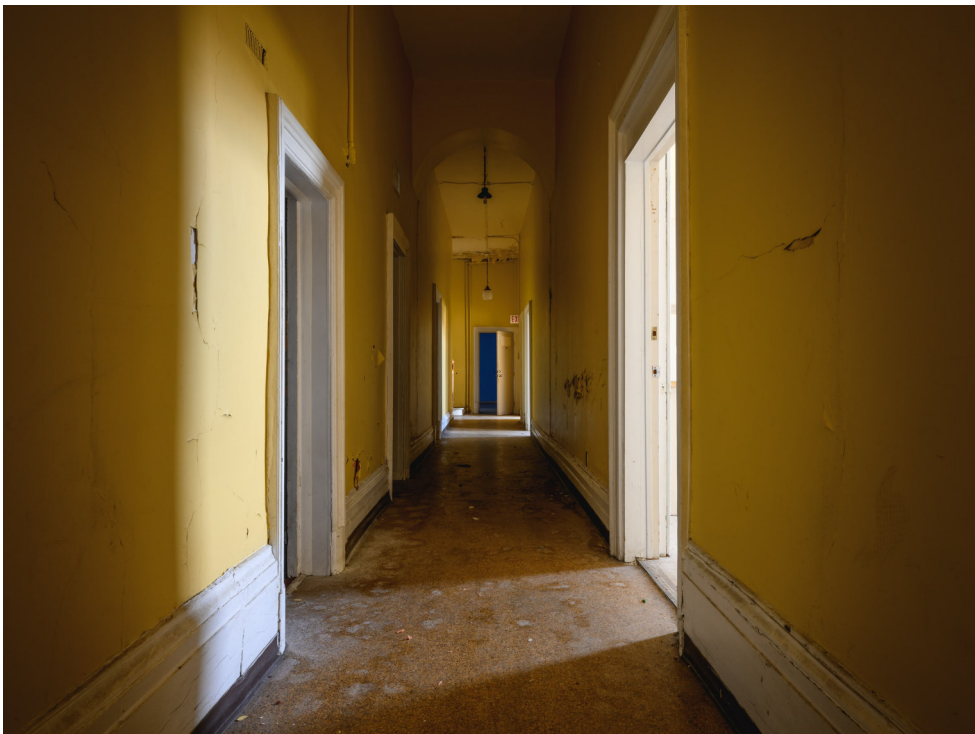
Figure 6.10 Historical Courthouse Ground Floor - Existing Conditions.
