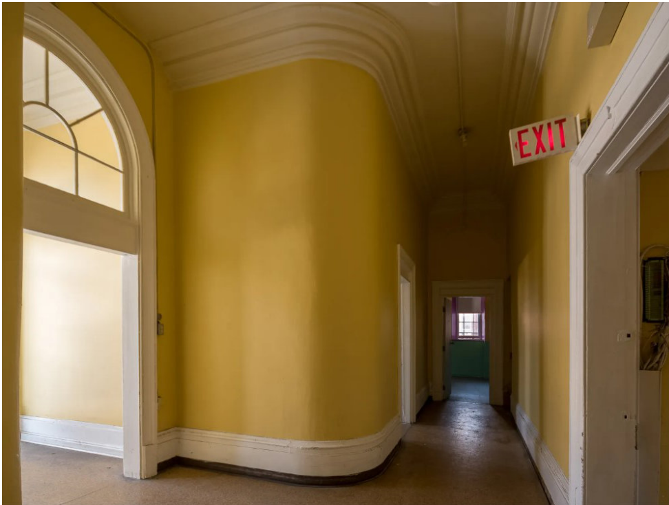
Figure 6.7 Historical Courthouse Ground Floor - Existing Conditions.
