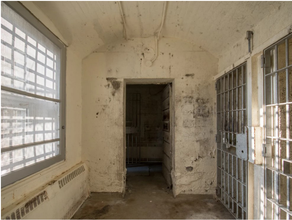
Figure 6.45 Interior view of the Jail Building Detail of vaulted ceiling.
