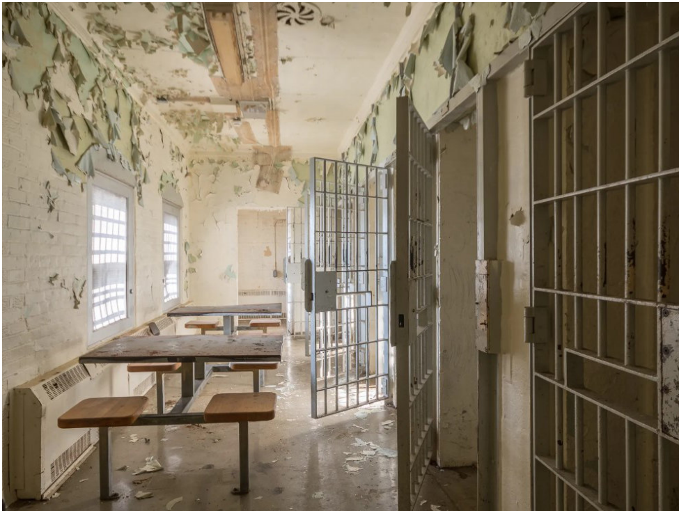
Figure 6.41 Interior view of the Jail Building Aisles adjacent to the cells.
