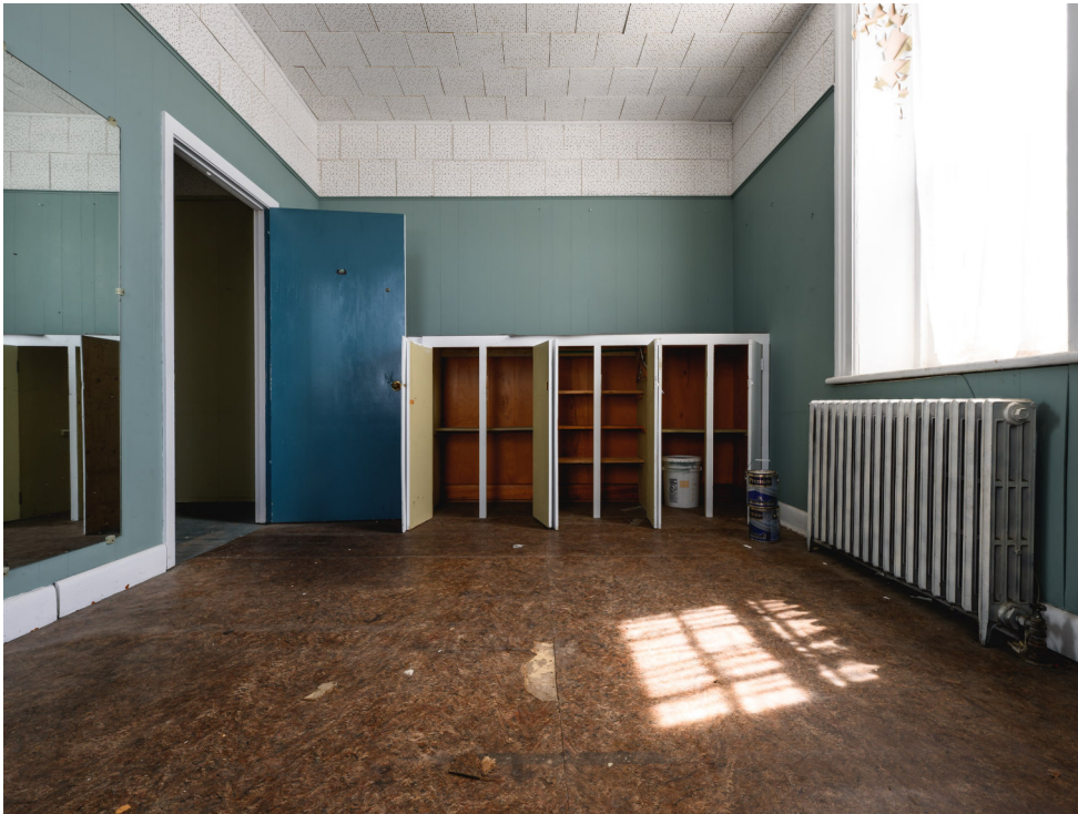
Figure 6.15 Historical Courthouse Ground Floor - Existing Conditions.
