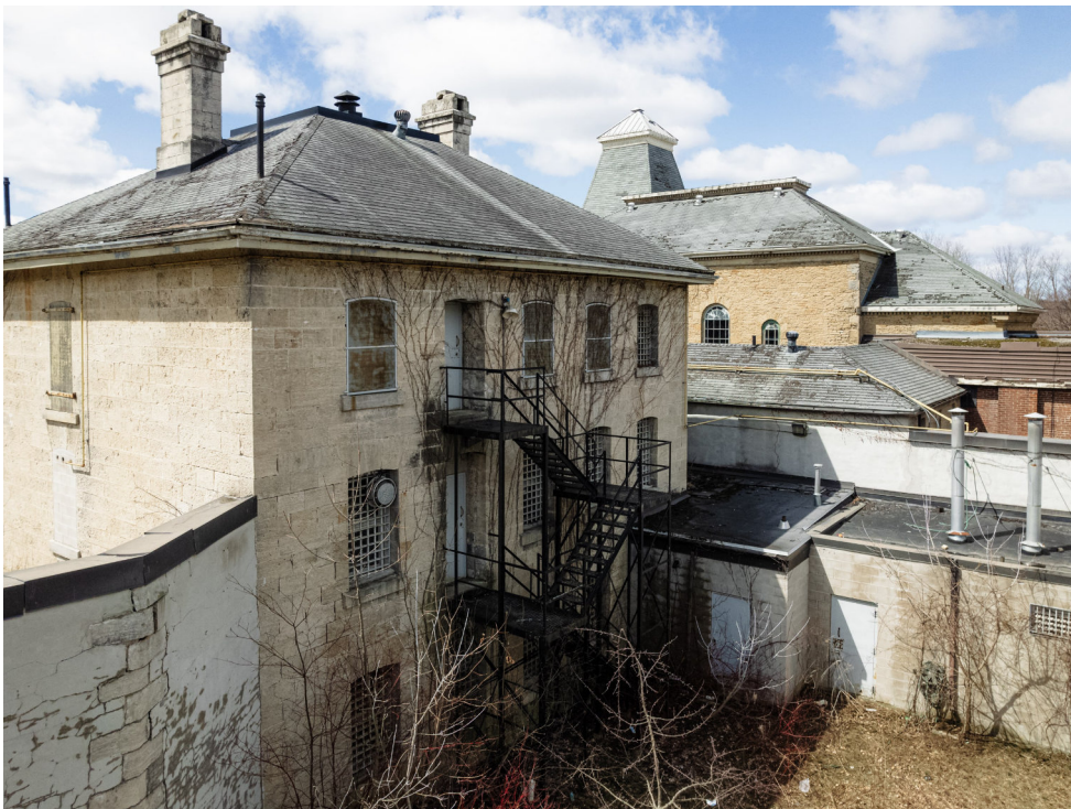
Figure 6.36 Birdseye view of the jail building viewed from the exterior yard.
