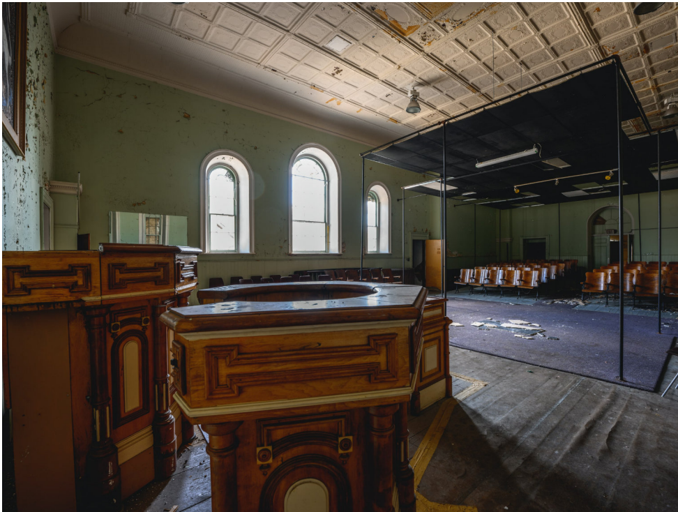
Figure 6.27 Historical Courthouse Interior view of the courtroom.
