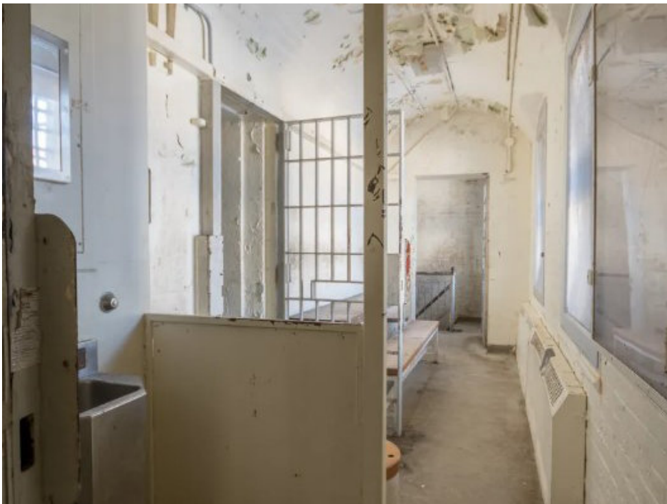
Figure 6.44 Interior view of the Jail Building Aisles adjacent to the cells.
