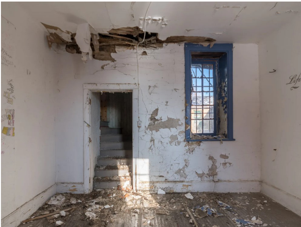
Figure 6.32 Historical Courthouse Access from the courtroom to the jail building through an internal staircase.
