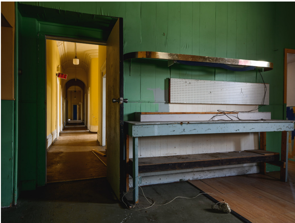
Figure 6.6 Historical Courthouse Ground Floor - Existing Conditions.
