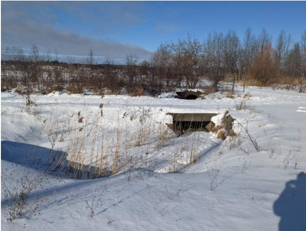
Photograph 1: View of the southern portion of the site, west facing. A storm water culvert leading into the site is visible (January 21, 2022).
