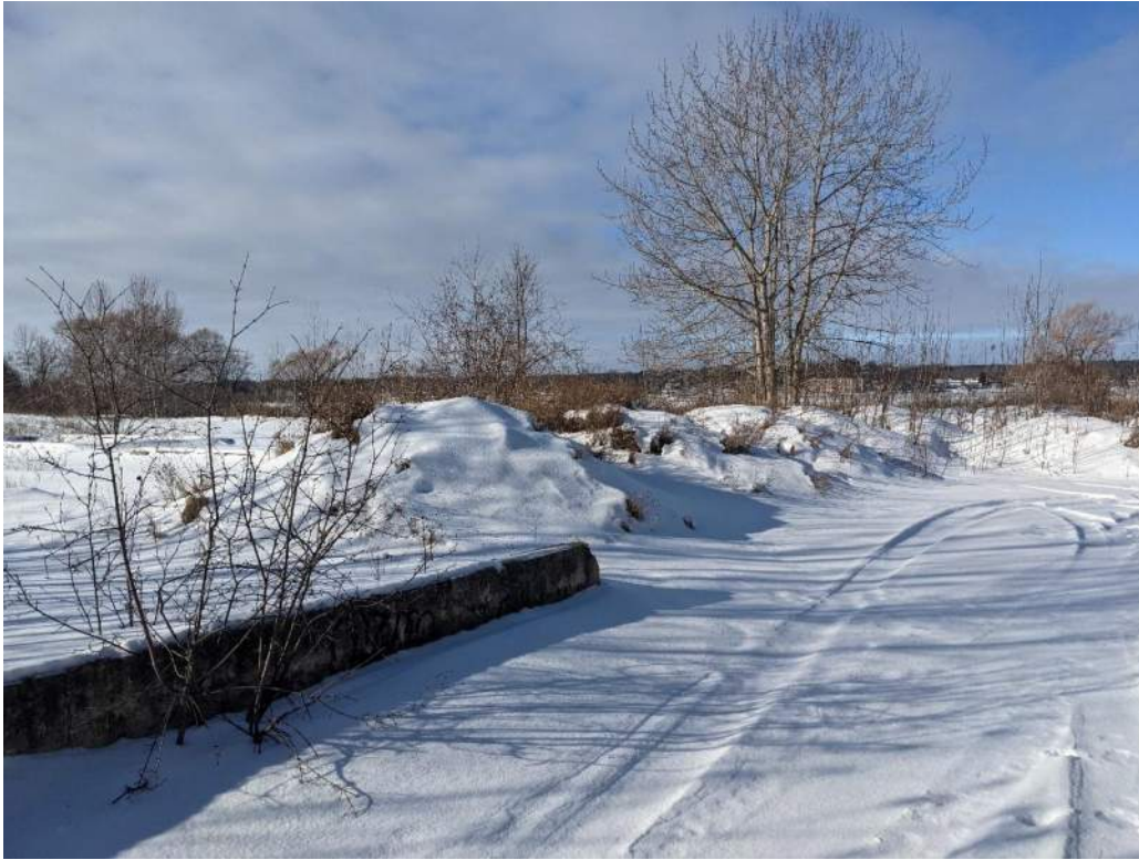
Photograph 3: View of the central portion of the site, west facing. Soil stockpiles with overgrown vegetation are visible (January 21, 2022).
