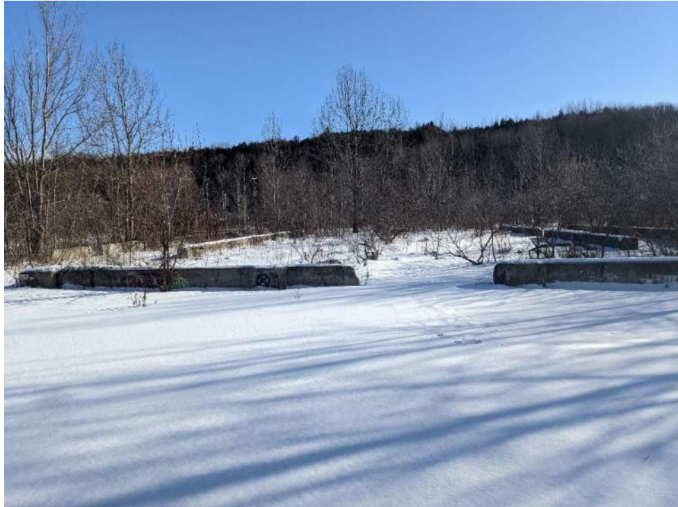
Photograph 6: Building foundations found on the northern portion of the property, facing east (January 21, 2022).
