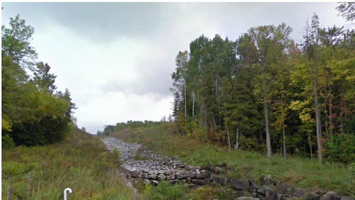
3 Kenny Drain, running east-west, adjacent to the southern property line.
