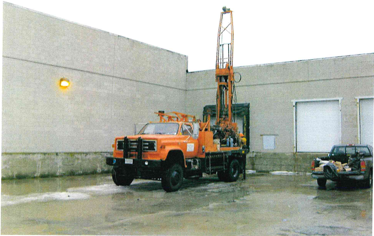
Photograph 1: View Southeasterly of Development of BH/MW1.
