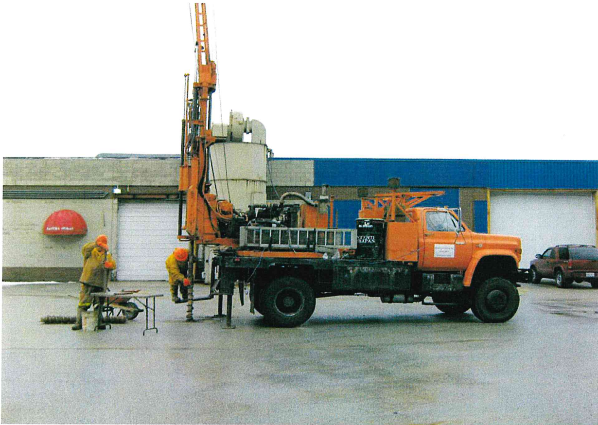
Photograph 5: Viewing Easterly of Development of BH/MW18.
