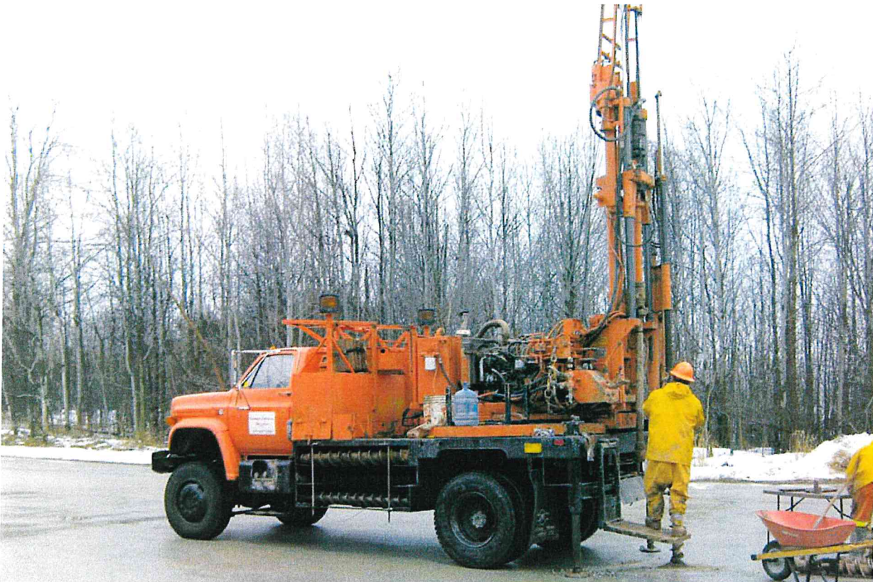
Photograph 6: Viewing Southwesterly of Development of BH19.
